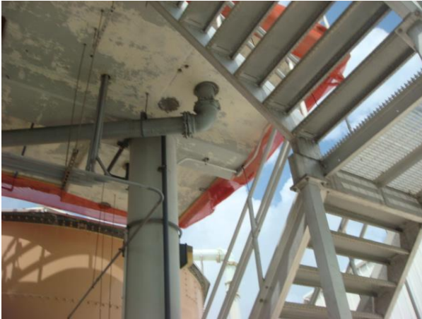
Incomplete concrete repairs.
