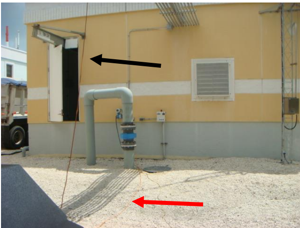
A long extension cord (red arrow) has been connected to an outlet on the exterior of the vacuum building to power the influent sampler. The outlet is also serving as the power source for the post-anoxic mixer (black arrow). The sampler and mixer cannot operate at the same time or the outlet will fail according to the operator.
