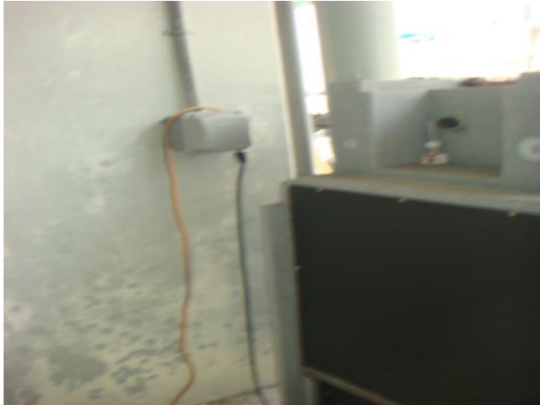
The outlet for power to the influent sampler was not operational at the time of the inspection.
